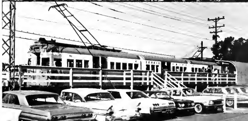
In the fall of 1964, the platforms were extended to accommodate the use of 88-foot-long articulated cars. All of the platform work was done with simple materials and plain design, in keeping with the minimal budget approach of a test project.
